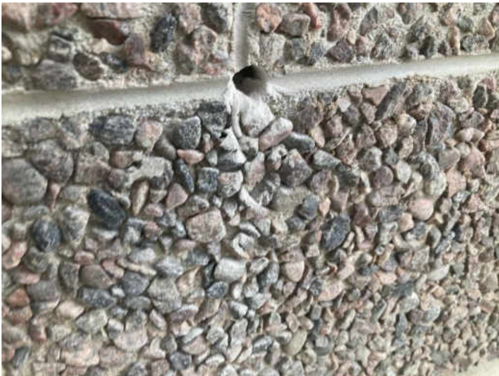
Wall, Vermiculite Investigation, Exterior (Location #: 3) no vermiculite overserved
